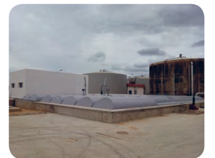
Example: Sewage treatment plant Badajoz / ES with BIOMOX ® CFR
