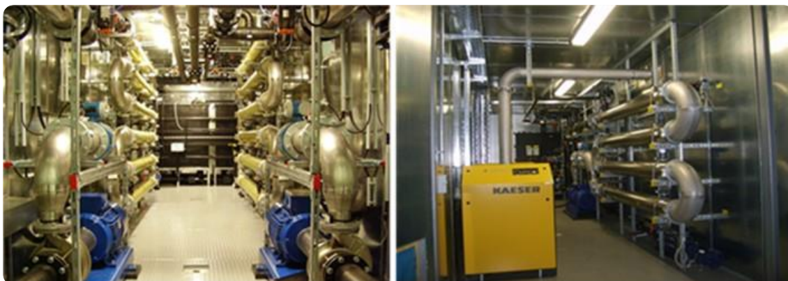
Picture 4: Inside of two UF containers. Left: two lines; right: one line
