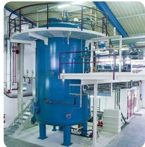
For example **TEXTILCOLOR AG, Sevelen / CH** – Wastewater treatment by using a BIOMEMBRAT® high-performance MBR with pressure biology for optimized oxygen transfer.
