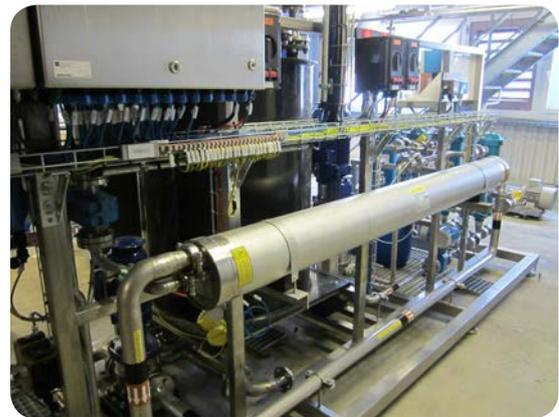
For example **Clariant, Gersthofen / DE** – The nanofiltration plant separates the nitrous additives from the process water to be disposed of separately and to save costs.
