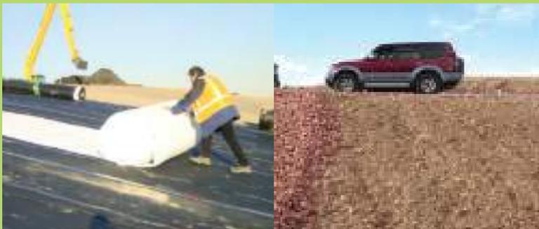
**Figure 19.5** Geosynthetic drainage mat (left) and drainage layer over a soil cap *Copyright Afvalzorg*
