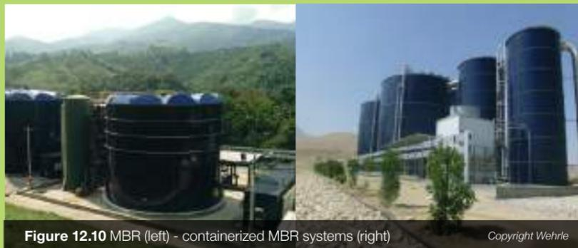
Figure 12.10 MBR (left) - containerized MBR systems (right)
