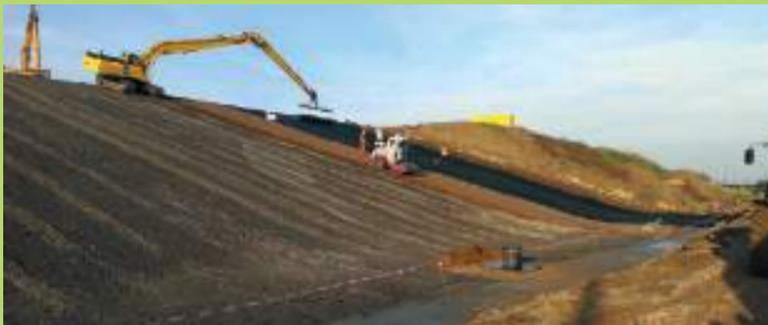
**Figure 19.6** Construction of a geomembrane over a geosynthetic clay liner *Copyright Afvalzorg*
