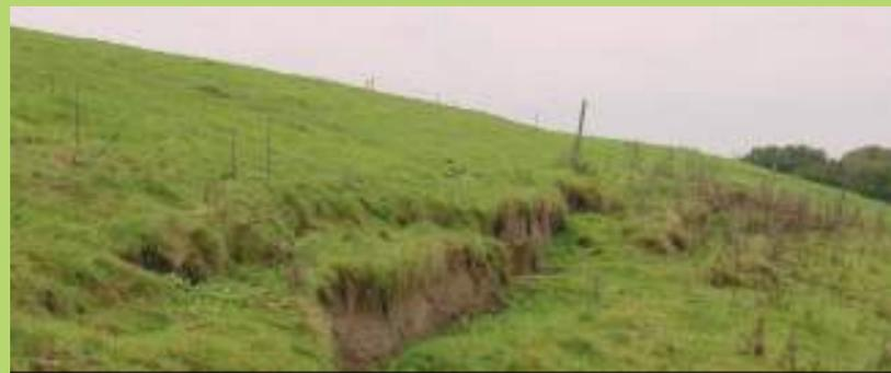
Figure 19.1 Damage of soil cover and barrier layer
