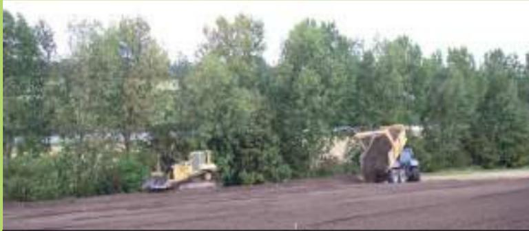
**Figure 19.4** Construction of a recultivation layer with a bulldozer *Copyright Afvalzorg*
