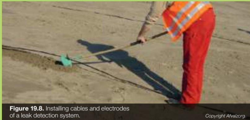
**Figure 19.8.** Installing cables and electrodes of a leak detection system.
