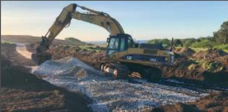
**Figure 18.2** Collection system below compost layer
