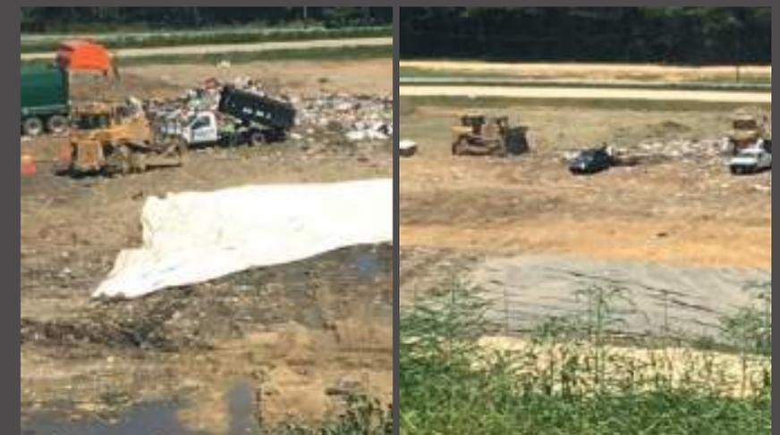
Figure 2.2. Application of Geotextile Matting
