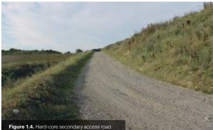
Figure 1.4. Hard-core secondary access road
