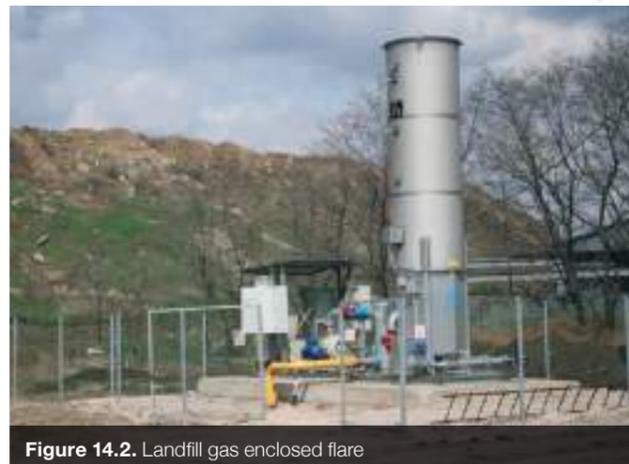
Figure 14.2. Landfill gas enclosed flare
