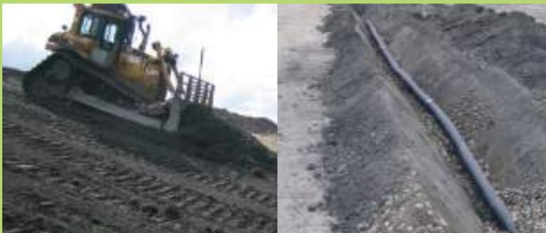
**Figure 19.7** Construction of a combined gas collection and foundation layer *Copyright Afvalzorg*
