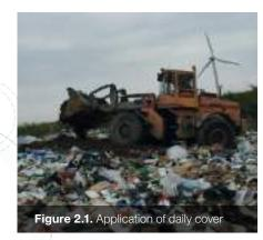
The most fundamental control to achieve good landfill performance is to regularly and completely cover the waste and to ensure it remains covered in all areas other than the active face, which should be kept as small as practicable.
