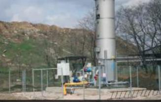
Figure 14.2. Landfill gas enclosed flare
