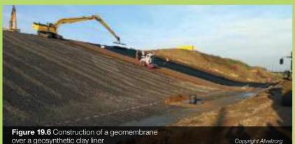
over a geosynthetic clay liner
