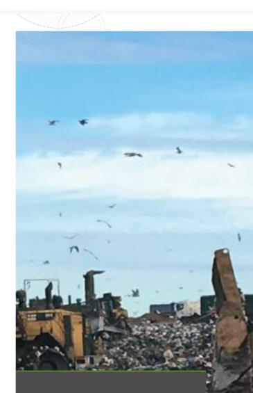
There should be sufficient space to allow trucks to unload at the foot or top of the working face as appropriate
