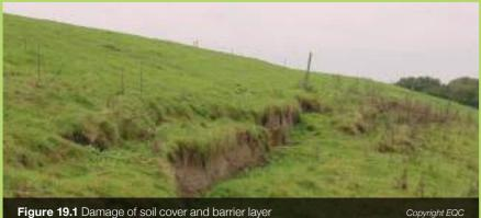
Figure 19.1 Damage of soil cover and barrier layer
