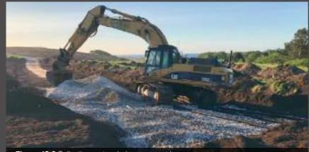
Figure 18.2 Collection system below compost layer
