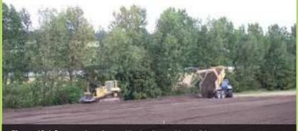
Figure 19.4 Construction of a recultivation layer with a bulldozer Copyright Afvalzorg
